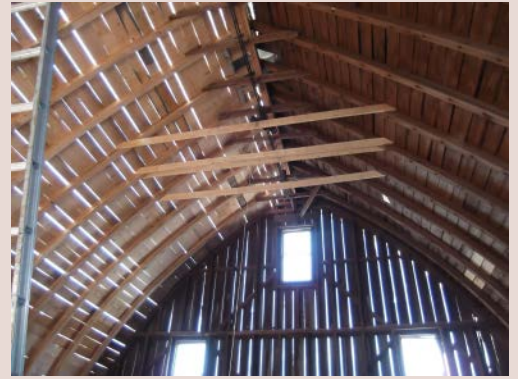
A patented truss system was used in the VanBenschoten barn. The original rafters are at right, the newly engineered side, meticulously reconstructed by Paul Waddington, is on the left.
