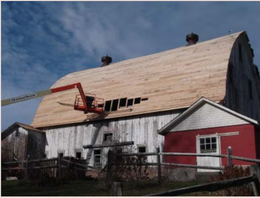
Preparing to close up the new roof on the barn Orson VanBenschoten built c. 1915.
