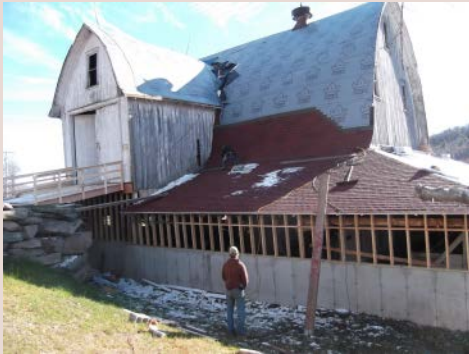
Jack Valek and crew did the difficult work of reshingling the gambrel roof. A new foundation has stabilized the hillside structure.
