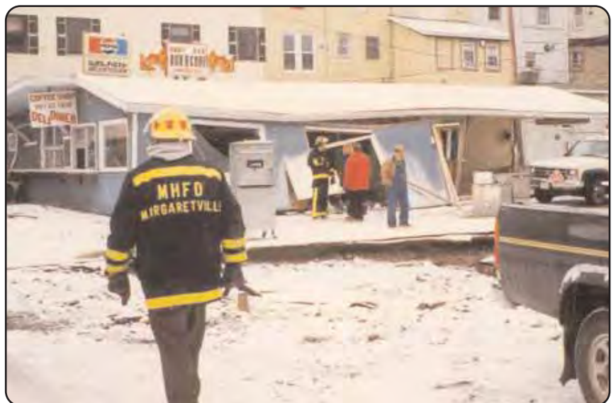
The Bun & Cone was demolished in the Flood of January 1996. It was rebuilt on an elevated concrete foundation and withstood the latest pounding from Irene.
